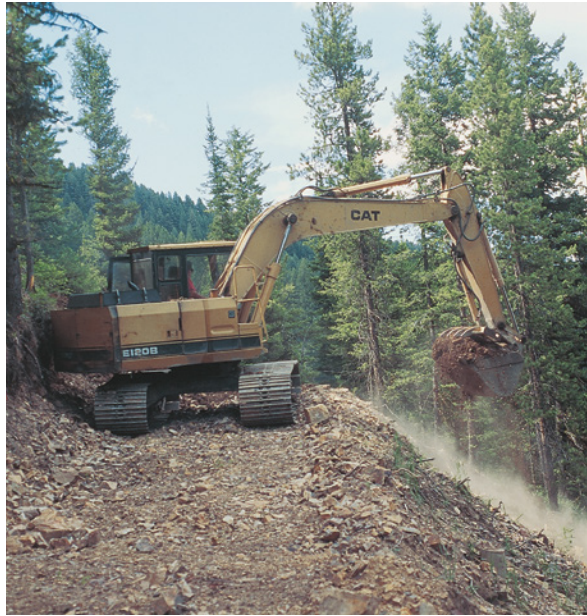
Excavator dismantling the road corridor.
