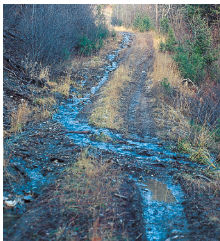
Not a major sediment problem yet — but when roads become channels for drainage, major sediment pollution can result.
