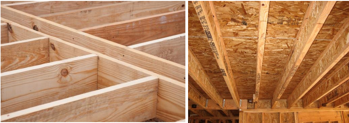
Figure 4.9: A) A standard wood dimension joist can range in size from 2 inches thick to 4 to 12 inches wide (photo credit Lampert lumber); B) Wood I-joists are manufactured on a linear basis, with no measurements for height and width. On average, an I-joist has a height of 11.75 inches and a width of 1.88 inches (photo credit APA – The Engineered Wood Association).
