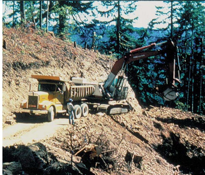
When constructing a full-bench road, the entire road surface is excavated in the hill. The excavated material is end-hauled, meaning the material is removed by truck to an area needing fill or to a stable disposal area.
