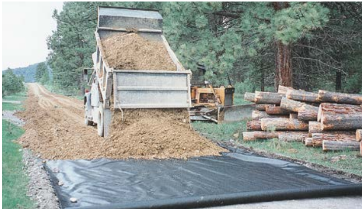
Geotextiles are used to reinforce subgrades by spreading the load across a larger area. This reduces the chance of settling and failure. It also allows road construction across wet areas, reducing the need to remove unsuitable roadbed material.
