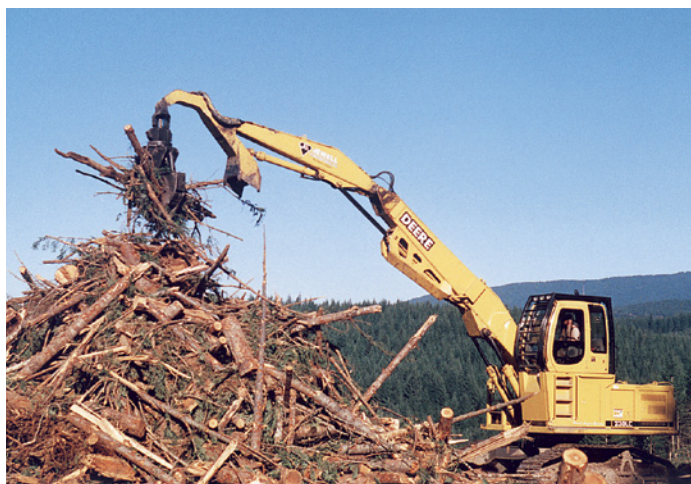
An excavator has the advantage of picking slash up rather than pushing it. Taller, more compact piles burn efficiently, with little soil disturbance.
