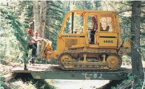
A portable bridge provides access across streams less than 10 feet wide, with minimal disturbance to streambanks or bed. Place portable bridges in locations with firm soil banks, level grade and minimal vegetation.
