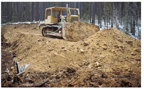
Cut-and-fill construction is common for gentle terrain. Soil is taken from cuts and pushed or "drifted" to where fill is needed to build up flat areas or cover culverts. Never let sidecast or waste material enter streams, and never place it in unstable areas where it might erode or slide into an RMA or within 75 feet of any stream.
