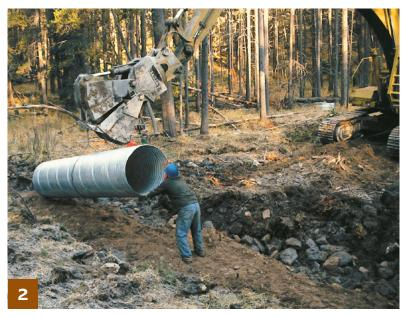
The culvert bed must conform with the natural streambed. The bed should be either rock-free soil or gravel. The culvert bedding should provide even distribution of the load across the length of the pipe. All stream crossings on Type F or Type SSBT streams must be designed to provide fish passage (see page 201).
