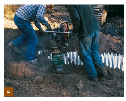
Tamping fill material throughout the entire backfill process is important. The base and sidewall material should be compacted first to reduce any chance of water seepage into the fill.
