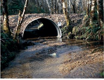
Arch culvert on a low-clearance road, sunk into the streambed to allow for fish passage.
