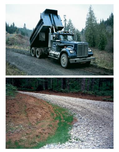
Road surfacing can double the cost of a road. However, gravel roads can provide all-weather access, reduce road maintenance costs and protect water quality by covering the soil with a weather-resistant surface.
