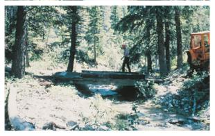
This 20-foot portable bridge was hauled on a flatbed truck and set into place in one day. The bridge cribbing that supports it is made from 10-foot-long timbers laid on the ground 4 feet from the stream bank.
