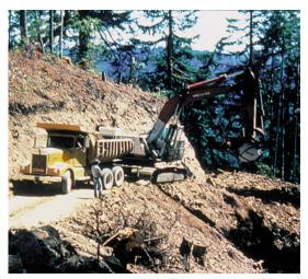
When constructing a full-bench road, excavate the entire road surface in the hill. The excavated material should be end-hauled. For example, it could be removed by truck to an area that needs filling, or to a stable disposal area.
