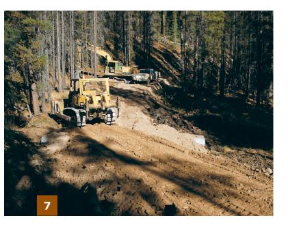
Layers of fill are pushed into place and carefully compacted to build up and maintain a consistent road grade. The crossing should be rocked to minimize the risk of sediment washing off the road and into the stream.
