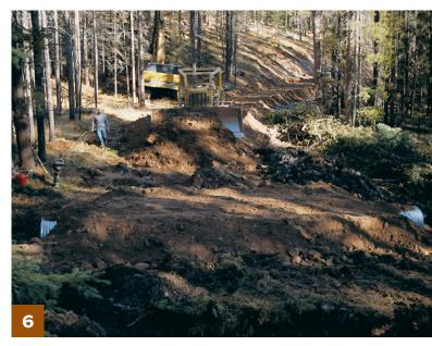
The road approach to the new culvert is the next phase of construction. Be sure that the culvert fill above the top of the pipe is at least 18 to 24 inches high to protect the pipe from damage by traffic.
