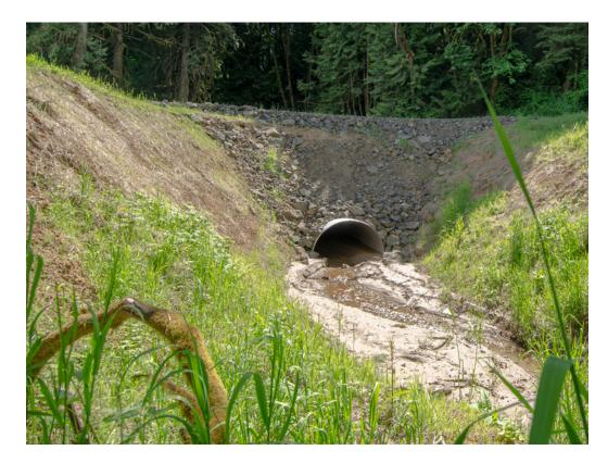
**Soil foundation**. Bedrock crossings may require bottomless arch culverts, bridges or fords.
