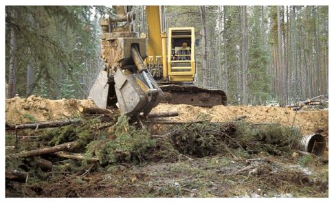
Slash-filter windrows are made of compacted logging slash installed along the base of fill slopes during road construction. Built by excavators, these 3-by-3-foot barriers are very effective at slowing surface runoff and keeping sediment from entering streams.
