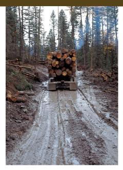
Roads receive heavy use during logging. Be aware of early signs of damage. Serious damage to road surfaces starts with excess water. Standing water is a sure sign of roaddrainage problems. Ruts indicate that road strength is deteriorating.
