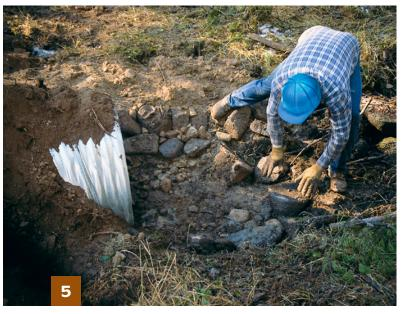
Armor the culvert inlet and outlet. Rocks, logs or grass seeding can be used to protect these locations against erosion. Check the area upstream and downstream from the culvert. Clear the upstream area of woody debris that might plug the culvert and place it at the downstream end.
