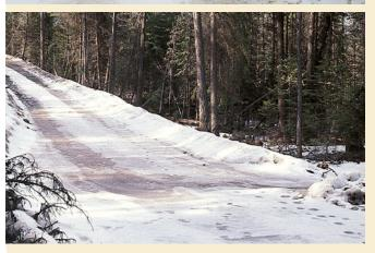
Snow berm breaks allow for drainage during snowmelt without damaging the road surface. They also serve as escape corridors for wildlife.
