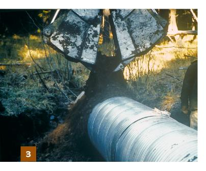
Secure each end of the culvert with backfill. Pour backfill material on top of the pipe. This allows finer soil particles to flow around and under the culvert sides. Larger particles roll to the outside. Fine soil particles, close to the culvert, compact more easily. Once the ends are secured by backfill, the center of the culvert is covered.
