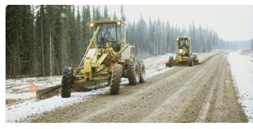
Slow, controlled grader operation is key to reducing culvert inlet and outlet damage. Reduce damage by keeping graders on the road running surface. Never side-cast gravel toward culvert inlets or outlets.
