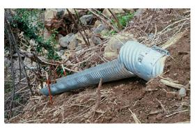
It may not always be possible to have the culvert extend beyond the fill. For steep fills, a half-round or flume should carry water beyond the fill.
