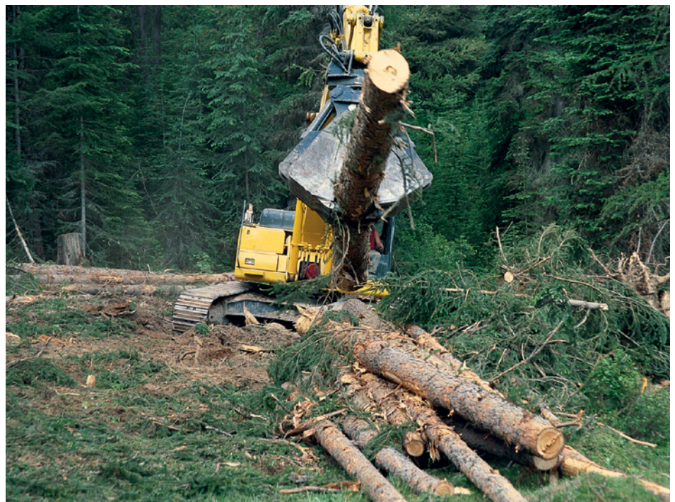
Excavators equipped with grapples are common choices for handling logs and doing other useful tasks during shovel logging.
